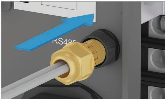
1. Unscrew the cable gland of the communication connection and remove the cable gland and seal.
