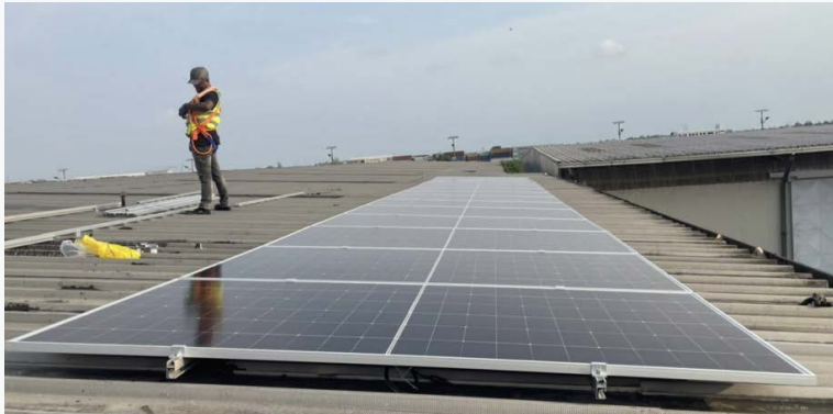
LONGi installs PV and energy storage equipment for the humanitarian emergency warehouse in Douala, Cameroon
