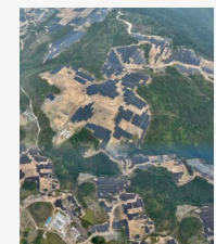
The 100 MW Photovoltaic Power Project in Rong'an County
